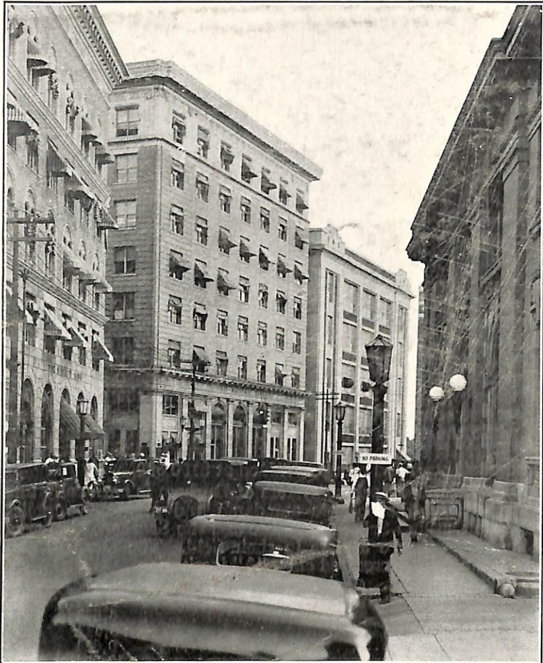
VIEW OF CORCORAN STREET, LOOKING SOUTH
